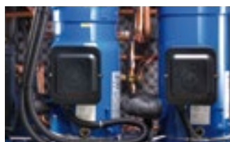
Higher energy efficiency and quieter operation thanks to scroll compressors.
